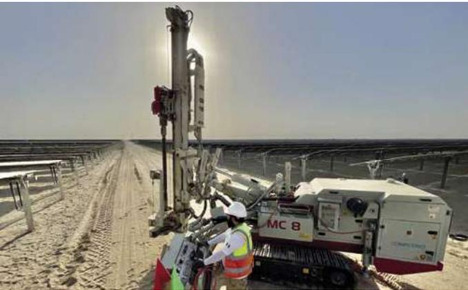
*One of the two Comacchio MC 8 rigs being used to install the foundations for a solar farm in the UAE*
