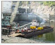
the first stage was performed using two concrete-drilling machines mounted on a concrete base and equipped with underwater lighting and video surveillance systems. Drilling was performed with underwater positioning of the machine by a diver using a floating crane. The hydraulic power pack on a barge was connected with the rig through high-pressure hoses. The machine was controlled by an operator on the barge with help from the images transmitted by the cameras.
