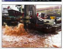
(DTH) hammer using an overburden drilling system. Three-metrelong canned rods of 273/530mm diameter, weighing 1,052kg each, have been specifically designed and manufactured for this project in the Czech Republic.
