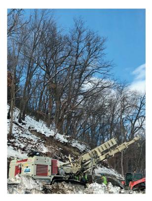
to a slurry/water drilling approach to equalise the head pressure during drilling and prior to removing the hammer and the drill steel from the temporary casing."
