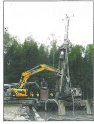
requests of Entreprenørservice and allow the use of casings of 813mm diameter. We also developed a new type of automatic down-the-hole (DTH) lubricator that facilitates the use of the DTH hammer. The machine features a variable-width undercarriage with adjustable hydraulic jacks, providing a wide, stable base for operating on the one side, and a narrow gauge that allows access to confined job sites on the other."
