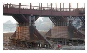
After installation, the new steel micropiles were then clad with wood to replicate the look of the bridge's original design
