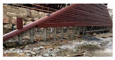
the installation of the new bridge foundations. At the same time, it allowed straightening of the bent bridge, bringing the deck back to its original height.
