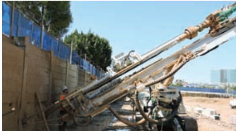
Here, the Comacchio carousel is only handling rods
