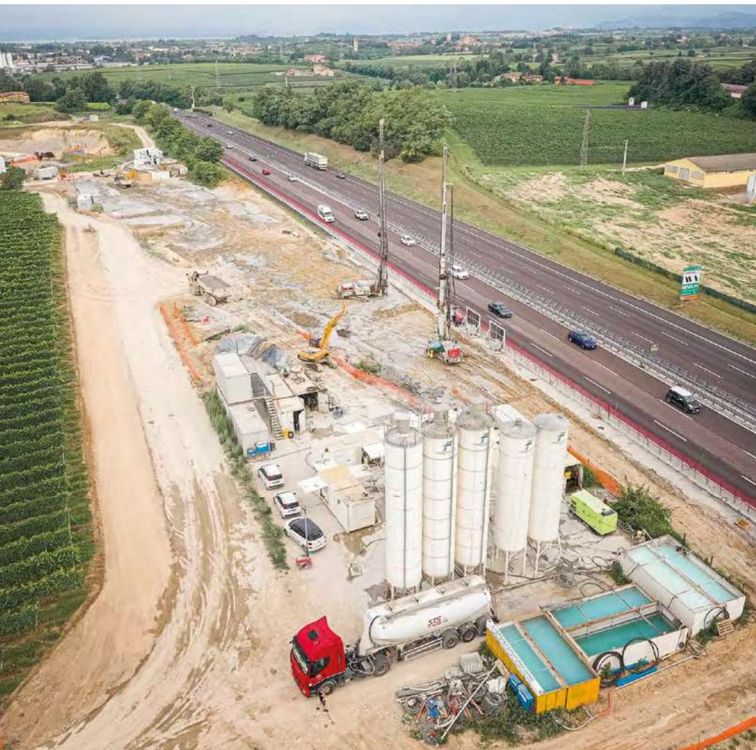
that communicates with the data-logger that equips the Comacchio machines. In this way, on-hole positioning is completely automated and extremely accurate, which would be impossible to obtain manually. The drilling and injection parameters are stored in the memory of the data logger, which automatically manages the injection phase for each individual column. The only thing the operator has to do is press a button."
