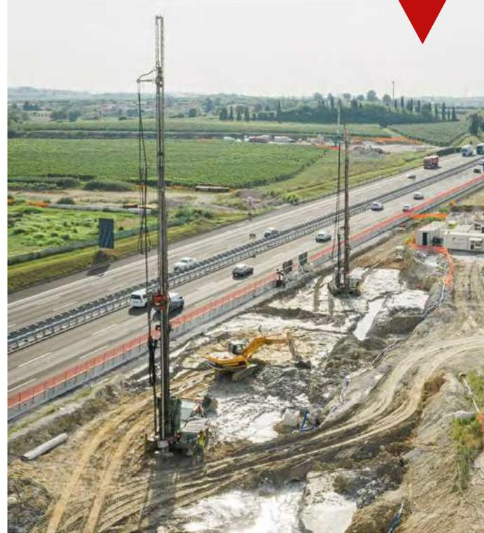
"In this way, we can work in an almost closed-loop system. After a pre-treatment phase with a desander that separates the coarse particles, the spoil goes through homogenisation tanks and finally ends up in the centrifuge, which separates both the cement and the remains of silt and clay. The dewatered cake is easily shovelable and can be loaded straight into a dump truck for disposal.
