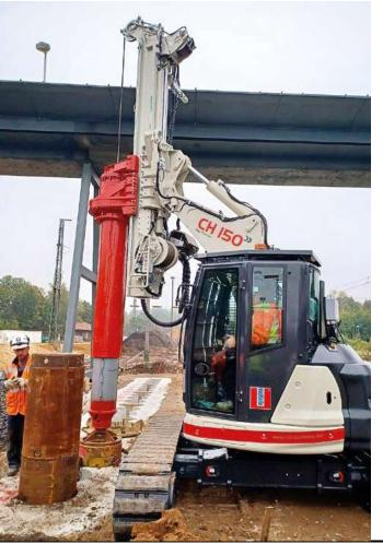
shared concept of hydraulic and electrical systems, electronically controlled through the CCS system (Comacchio Control System – a user-friendly control software entirely designed by Comacchio, controlling all drilling parameters and allowing for the complete management of the machine, including fault diagnostics). The advantages that this consistency offers are significant, both at the operational level and in terms of after-sales assistance.
