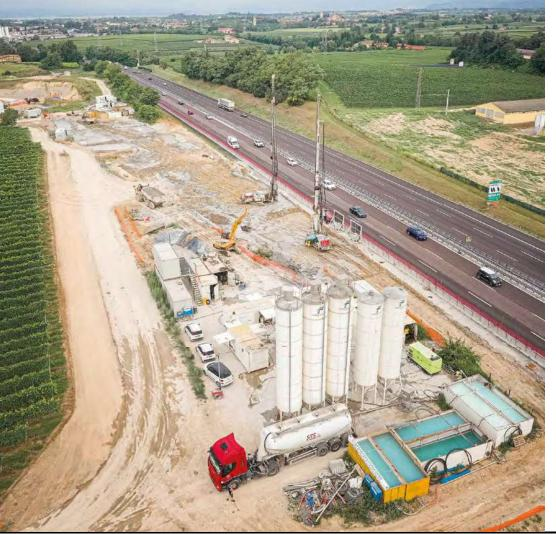
on the Southern side of the A4. The project involves consolidation works for the excavation of the 3.7km long San Giorgio tunnel which will cross the A4 motorway near the municipality of Sona, not far from Garda Lake. The consolidation is carried out with the help of vertical jet grouted columns that are installed from the surface ahead of the excavation face, for a total length of about 400m.
